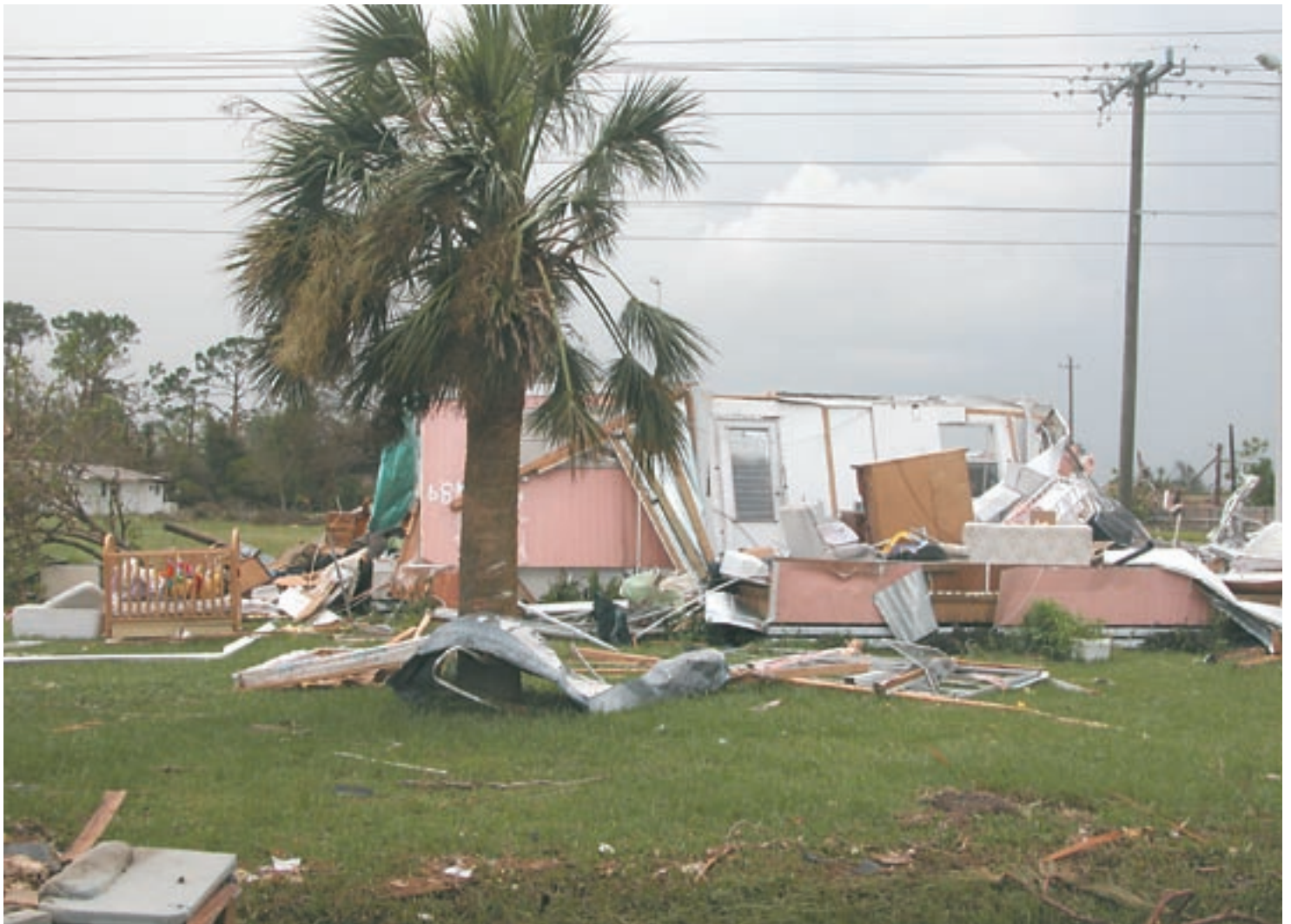
Manufactured housing cannot withstand Category 4 winds like those of Hurricane Charley. Photos courtesy of John Holmes.
